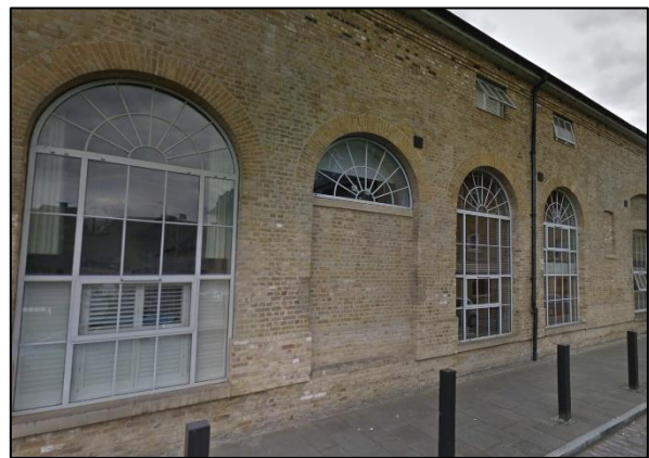
The former Goods Shed has been redeveloped
