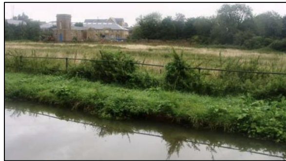
London Road/Viaduct Road junction: an important gateway to Ware
