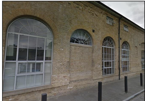
The former Goods Shed has been redeveloped
