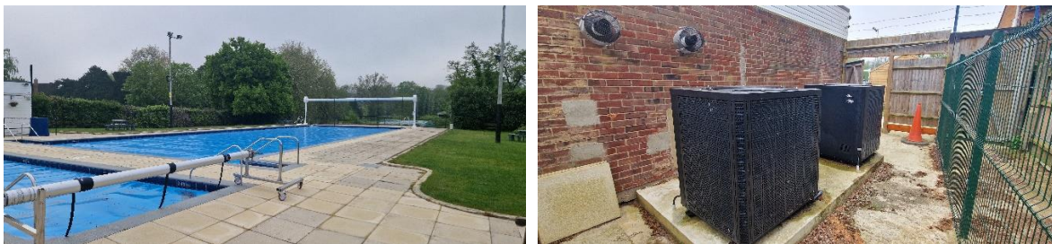
New Lido pool and Air Source Heat Pumps
